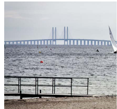
The Øresund Bridge
