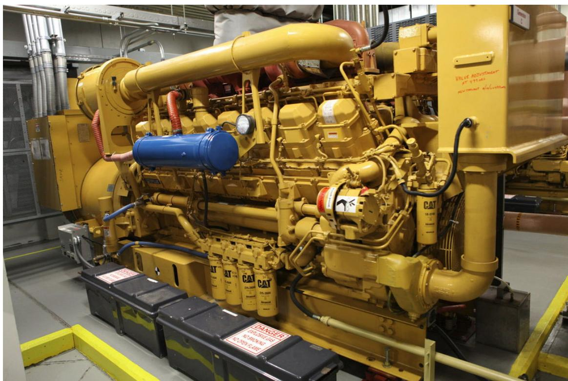
**LOW-TECH AMID HIGH-TECH** *A backup diesel generator at a large computer data center, one of six in the room. Combined, they could provide enough power for a community of 7,000 homes. Richard Perry/The New York Times*
